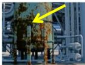
That tank looks rusty and corroded!
