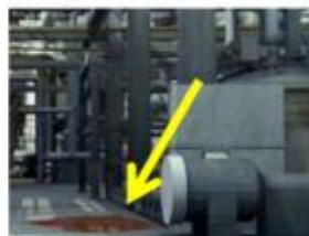
What is that puddle on the floor?
