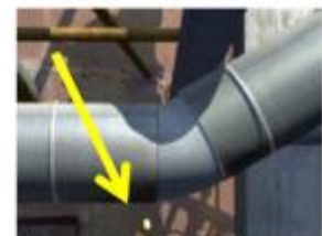
Is something dripping from this insulated pipe?
