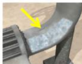
Is that a crack in this pipe?
